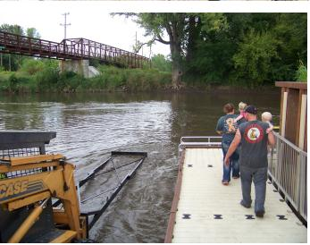
This shows how FPRF has cleaned the mud sediment from the boat launch at Tutty's Crossing. A twenty foot long pusher blade is attached to a skid-loader to push the sediment off the ramp, into the river. Works well!
